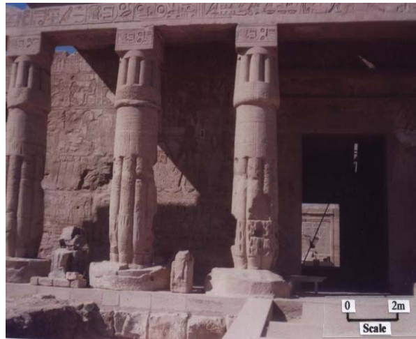
Figure 6: Moderately weathered East facing wall side of the Temple (parts of investigation numbers 5 and 6).
