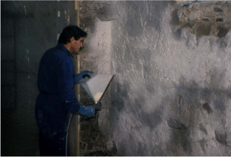
Figure 10: St. Georgen, salt reducing treatment
