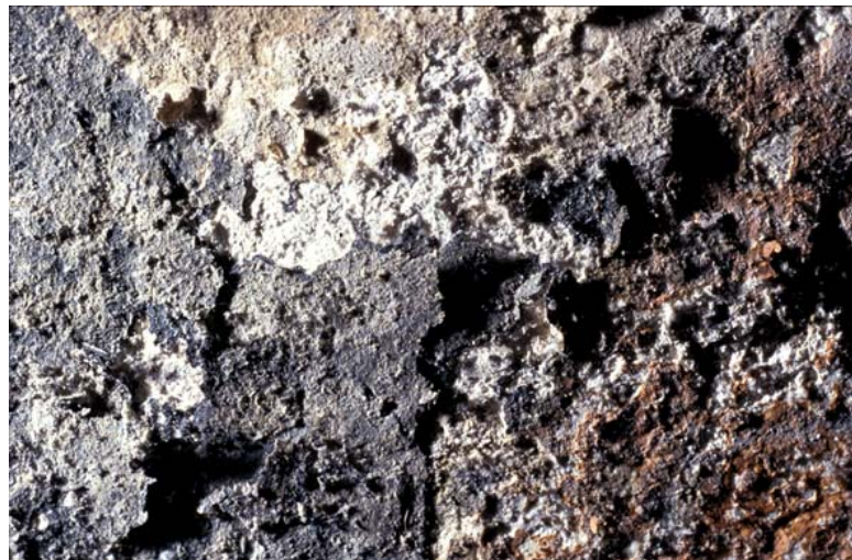
Figure 12: St. Georgen, scaling of the paint layer by the dynamic of salt crystallization
