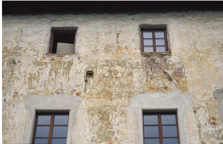
Figure 2: Facade paintings of Parz, the covering of the paintings by limewash, during the counterreformation (around 1600) was meant as destruction, but acted as protection layer. Because of lack of maintenance the covering limewash layers have been partly fallen off by the weathering activity exposing the paint layer. The dark areas indicate a heavy sulfatation.
