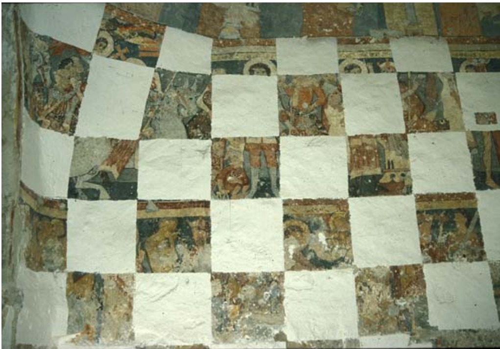
Figure 11: St. Georgen, during the removal of the salt reducing poultice
