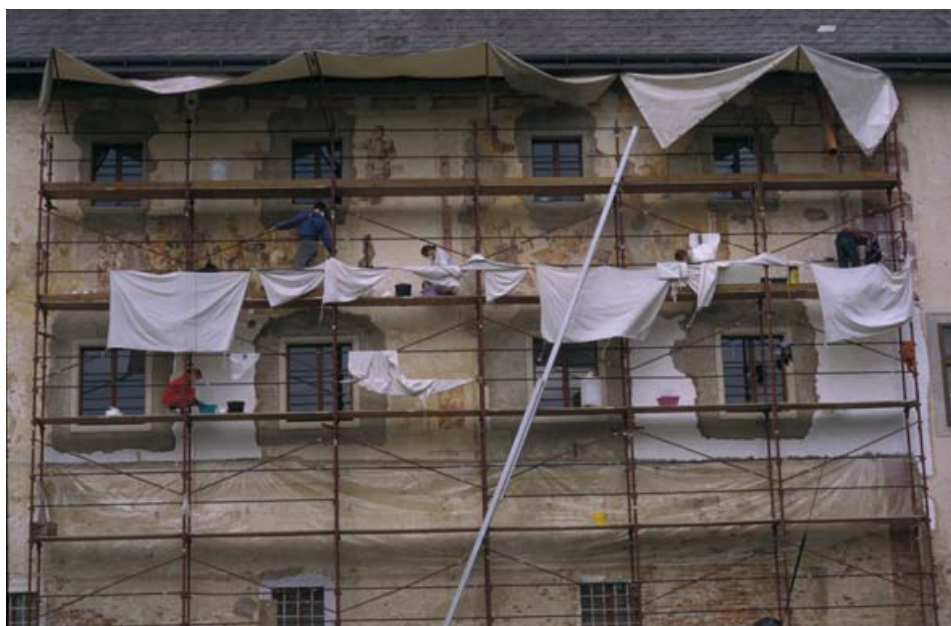
Figure 5: Facade paintings of Parz, during the application of the Florentine treatment
