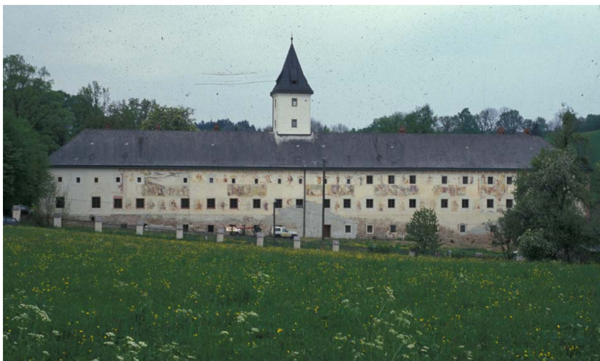
Figure 6: Facade paintings of Parz, general view after the treatment of the remaining painted areas
