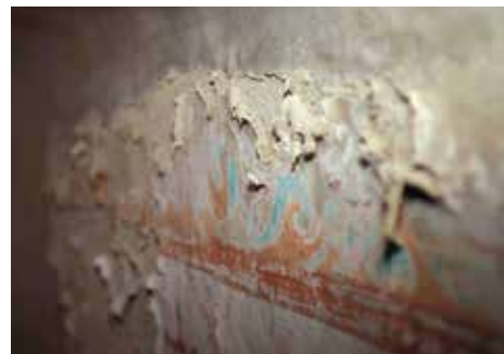
Figure 2: Salt-induced flaking or exfoliation of the wall paintings in Cave 85
