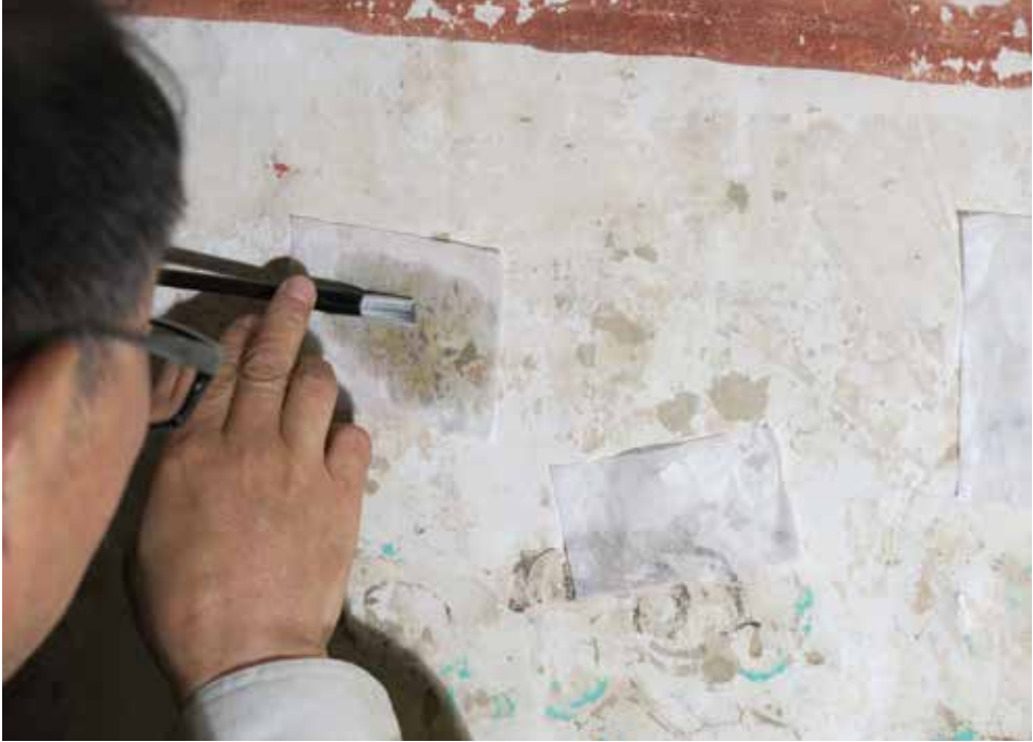
Figure 8: Relaying of exfoliated areas was undertaken with water and water: ethanol mixes applied with brushes through paper tissue.
