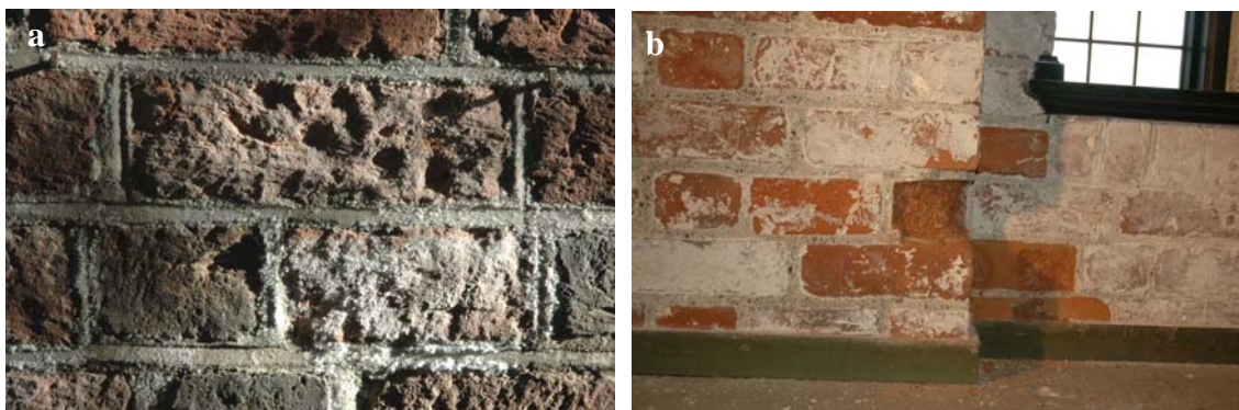
Figure 1. (a) Harmless salt effluences at the surface of non plastered brick masonry from where the salts can be removed by use of a brush. (b) Material damaging subeffluences (salt crystallization inside the pores).
