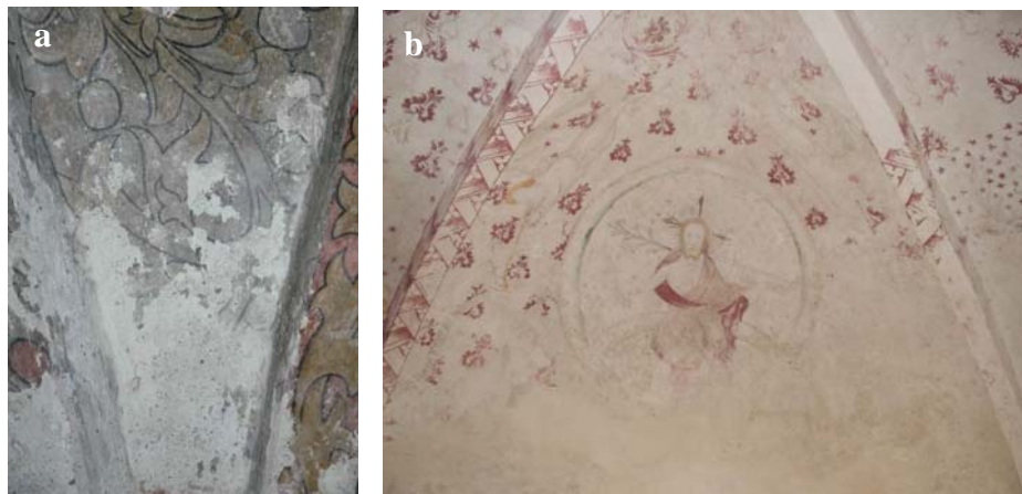
Figure 3. Salt induced deterioration of murals (a) From a monastery vault (b) From a church vault.
