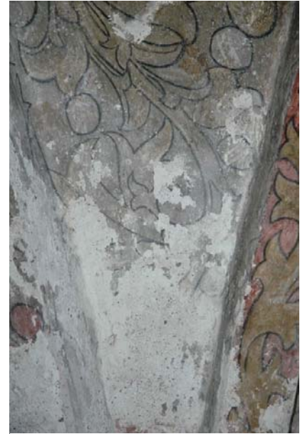
Figure 4. Deterioration of the murals in the Carmelite Monastery in Helsingør, Denmark.
