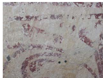
Figure 3. Close up of a partly deteriorated mural. Rørby Church, Denmark
