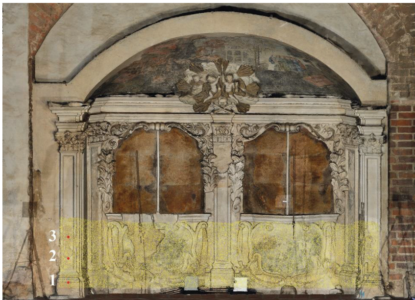
Figure 2: Baroque tomb, moisture and salt damage (highlighted in yellowish) in the lower area of the tomb, on the left are marked the drill powder extraction points for the quantitative analyzes in one height and three depth profiles
