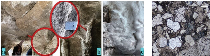
Figure 3: a. Seepage is seen near a fissure in the roof, b. Typical deterioration pattern on no fissures area, c. North wall in Cave 4 has been weathered to tafoni
