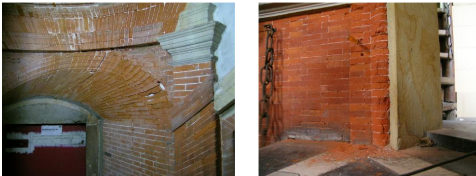
Figure 2. (left) Salt crystallization damage on one of the masonry masterpieces Figure 3. (right) Selected test area (internal wall of the tower at the 1 st floor)
