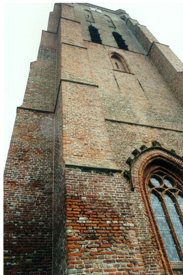
Figure 1: Tower of the church of Oostkapelle
