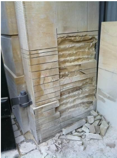
Figure 1: Removal of experimental stone pieces from wall
