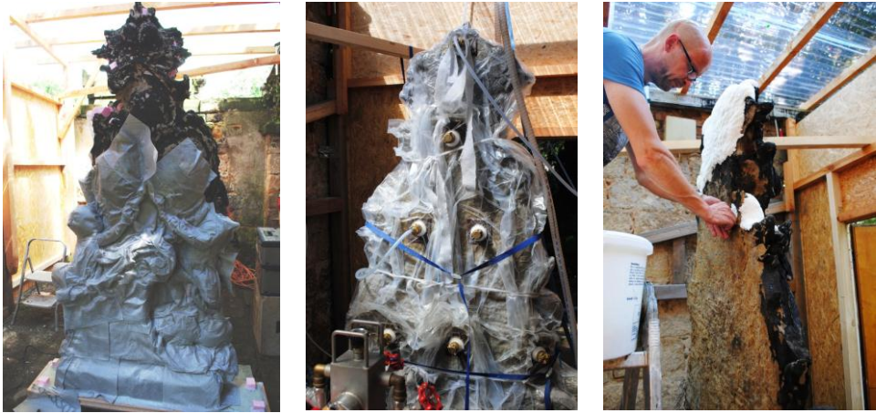
Figure 3: The object during the desalination procedure: Protecting the sandstone surface by permeable textile gauze (left), 'vacuum' desalination in progress (middle), and final application of cellulose poultice (right).
