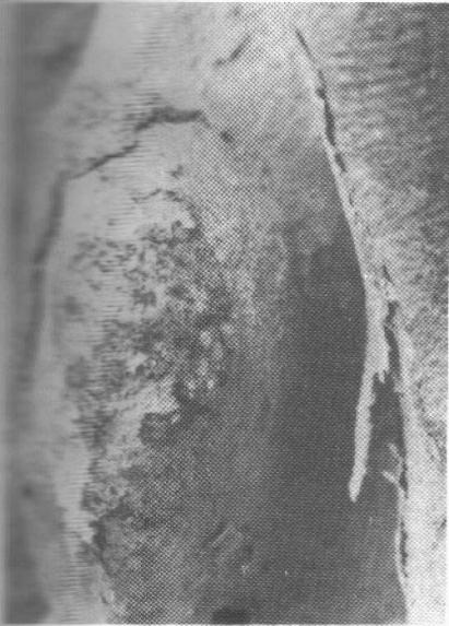
**Fig. 2A** – Detail of the salt decay near base of statue of Figure 1A.
