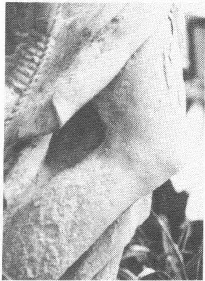
**Fig. 2B** – Detail of salt decay of statue of Figure 1B.
