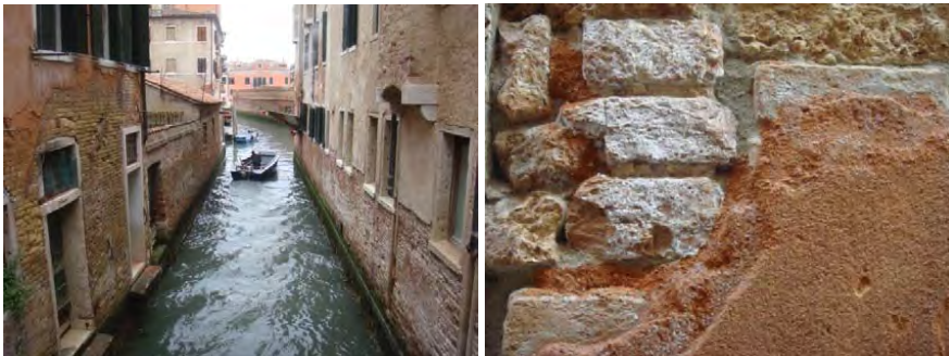
Figure 1.1: Examples of the damage to brickwork in Venice. The buildings in Venice are in a constant state of destruction almost entirely due to marine salt (dominated by NaCl).
