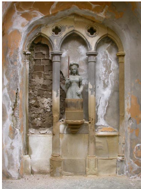
Figure 1: The metallic sculpture of Joan of Arc resists salt crystallisation while sandstone archery and lime rendering deteriorate at the garden wall of Stolzenfels Castle.
