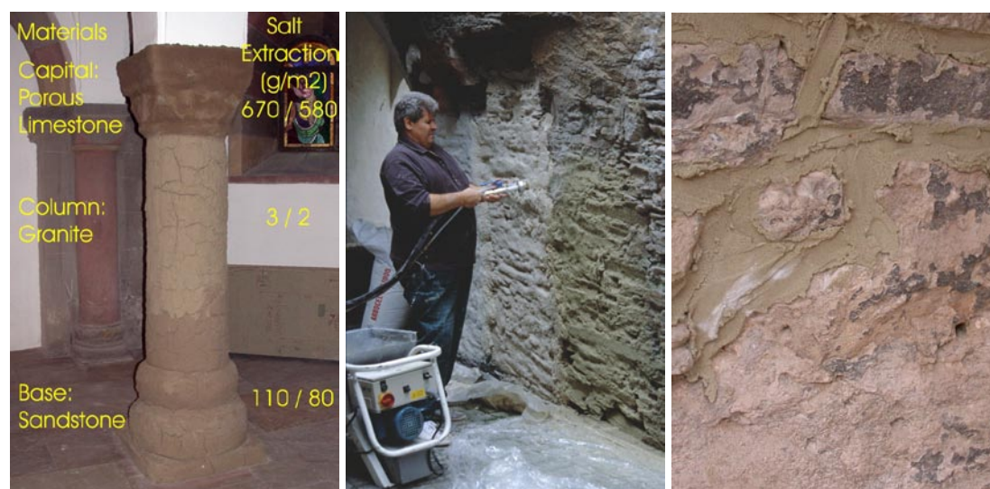
Figure 7 (left): Salt reduction at a column in the crypt of the church of St. Goar. Numbers show the amount of salts extracted by the first two cycles of bentonite poultices.
