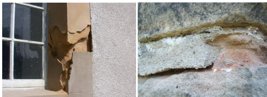
Figure 15 (left): The wall is covered with a water-repellent rendering, deteriorated parts of the sandstone elements had been replaced by dense cementitious mortar. The sandstone frame is the only place where water can evaporate, so transport of water and salt is redirected into the sandstone. Severe damage is the result of the high concentration of salt in the sandstone.
