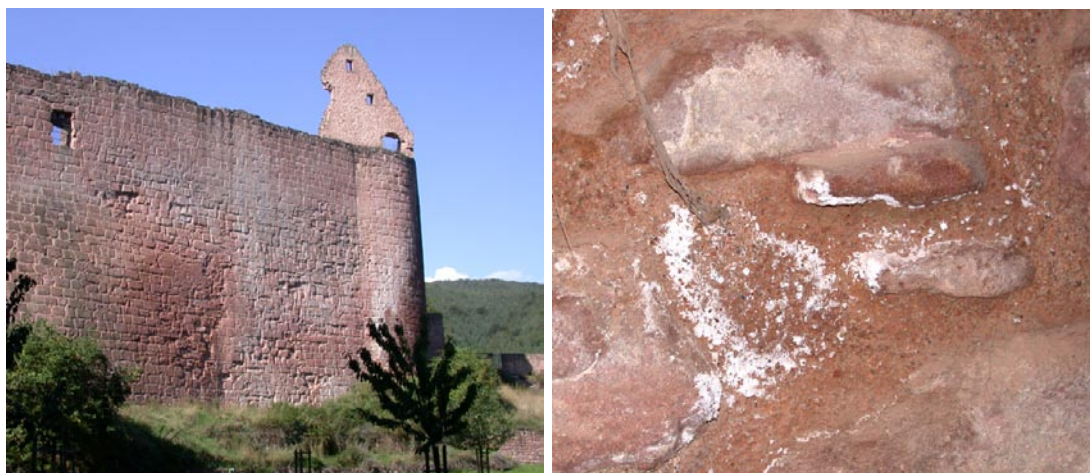
Figure 17 (left): Sandstone wall from Hardenburg Castle with salt efflorescences and hygroscopic moisture stains.
