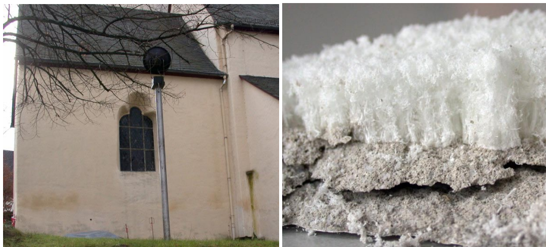
Figure 13 (left): Humidity and salts ascend behind a cementitious renovation rendering and now have reached the zone above the newly rendered basal zone.
