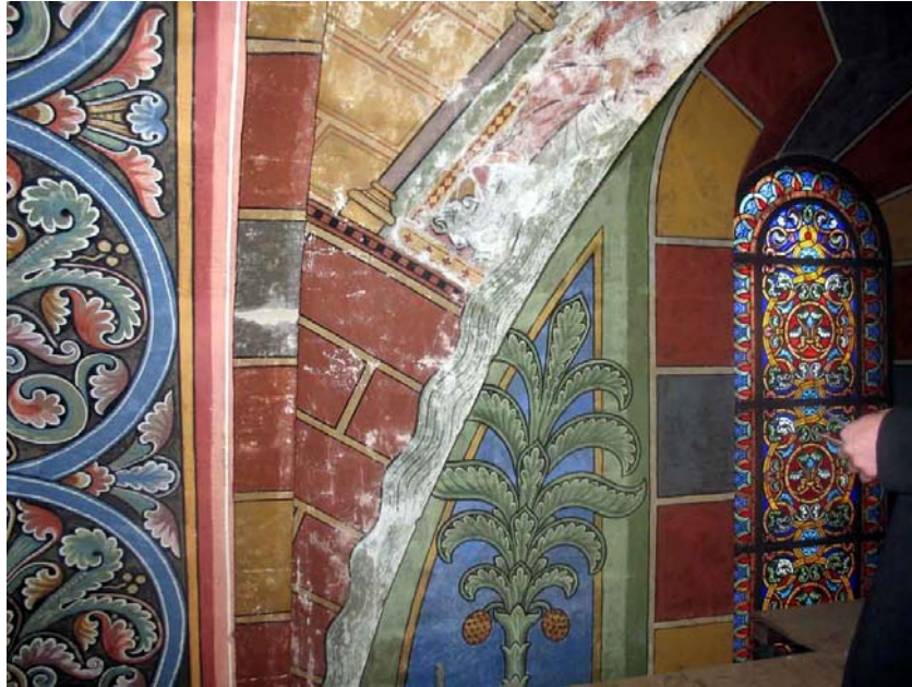
Figure 1. Salt damage of the wall paintings in the cathedral in Königslytter
