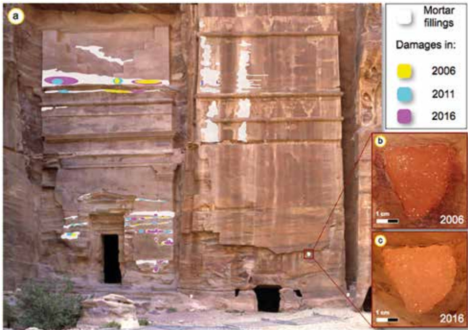
Figure 4: a) Ongoing damage progress of restored areas treated with silica-sol mortars during a period of 15 years on monument 825. b) Sample of a dry-slaked lime mortar just after application in 2006 and c) after 10 years.
