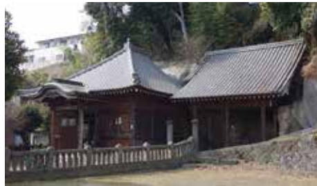
Figure 2: Exterior of the shelter
