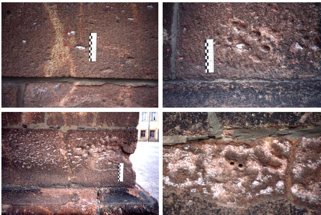
Figure 4: Stages of the development of alveoli at the church St. Kunigunden in Rochlitz: Weathering out of single lapilli components (above). Smaller pits can coalesce to bigger alveoli (lower left), salt efflorescence is always present. Further salt weathering forces the formation of a system of holes and ridges (lower right, with the drill holes for detailed salt investigations).
