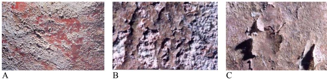
**Figure 4 A-C:** Hardham Church, West Sussex, England: Detail of wall paintings: showing damage due to salt crystallisation and organic coatings (photo: A. Heritage, Conservation of Wall Painting Department, Courtauld Institute, 1994)
