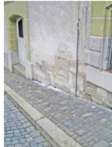
Figure 2: Left: Belfaux (canton de Fribourg, CH), north façade of the Lanthen-Heid manor (1526). The damages that affect the render and the underlying molasse-sandstone are mainly the result of splashing traffic along this street (3.09.2008). Right: Lausanne (canton de Vaud, CH), rue Saint-Etienne (20.01.2010). During dry winter cycles the residues of recrystallized deicing salts can be seen at the foot of façades that can either be mobilized and suspended in the air or enter the material when dissolved in water via hygroscopicity, rain, or more snow.
