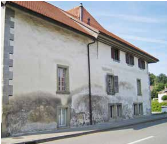
Figure 2: Left: Belfaux (canton de Fribourg, CH), north façade of the Lanthen-Heid manor (1526). The damages that affect the render and the underlying molasse-sandstone are mainly the result of splashing traffic along this street (3.09.2008). Right: Lausanne (canton de Vaud, CH), rue Saint-Etienne (20.01.2010). During dry winter cycles the residues of recrystallized deicing salts can be seen at the foot of façades that can either be mobilized and suspended in the air or enter the material when dissolved in water via hygroscopicity, rain, or more snow.
