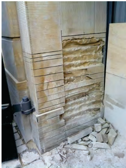
Figure 1: Removal of experimental stone pieces from wall
