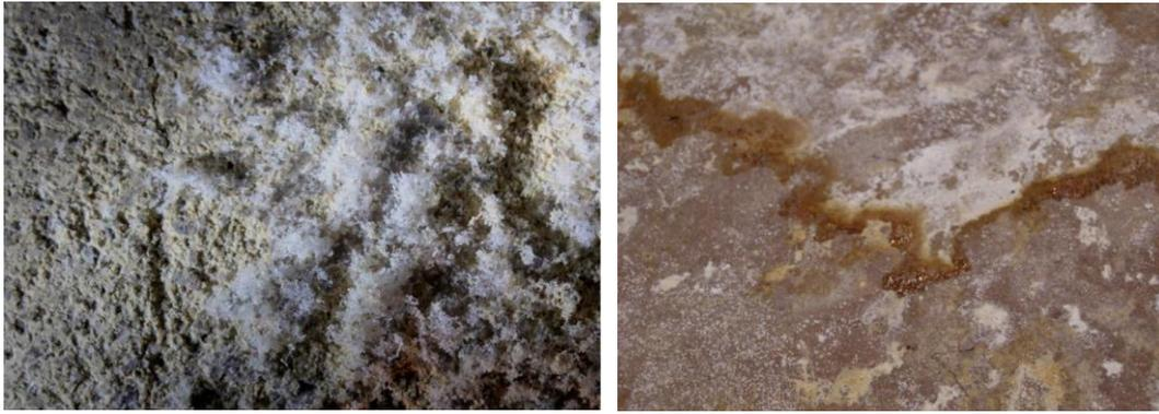
Figure 4. Macro photos of the white salt efflorescence (left) and brownish stain (right).
