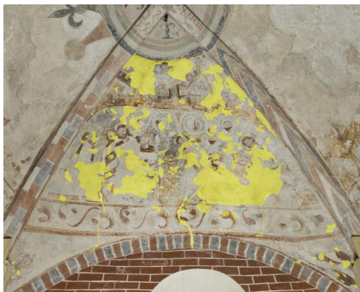
Figure 2. Areas of the north web where the pictorial substance is missing are mapped in yellow.
