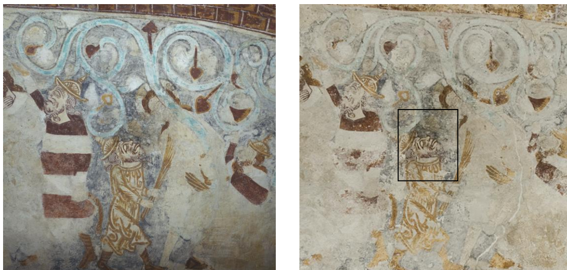
Figure 1a and 1b. Condition of the north web of the chancel vault in 1984 (a) and 2009 (b). Rectangle on 1b marks area consolidated with acrylic dispersion in 1984. Photo: Roberto Fortuna.
