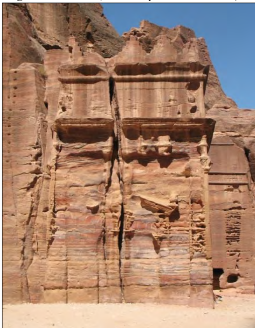
Fig. 1.3: Weathering damage on Tomb No. 70.
