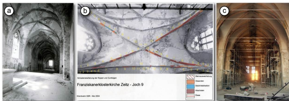
Figure 3: a) The church before conservation. b) An exemplary mapping of damages of the ribs of vault no. 9. c) The church during conservation. In the front the first restored vaults are visible.
