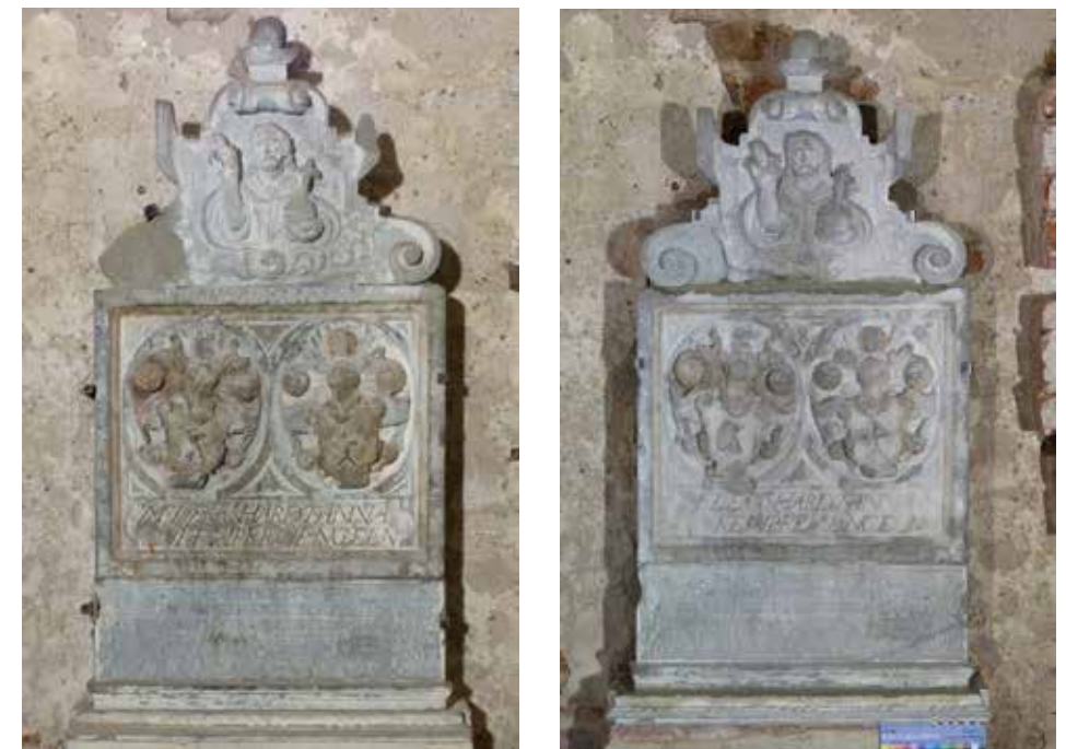
Figure 7: Epitaph of Leonhardt Kämpfe in Werben before (left) and after conservation (right)
