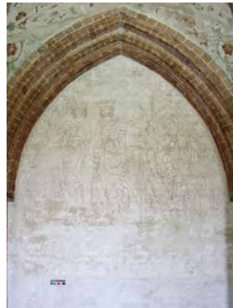
Figure 3: After the application of desalination poultices
