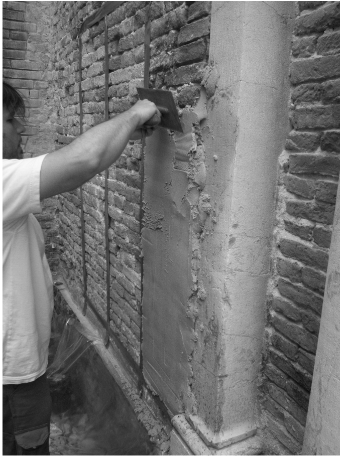
Fig. 1.2: An example of poultice application on a test wall in Venice.
