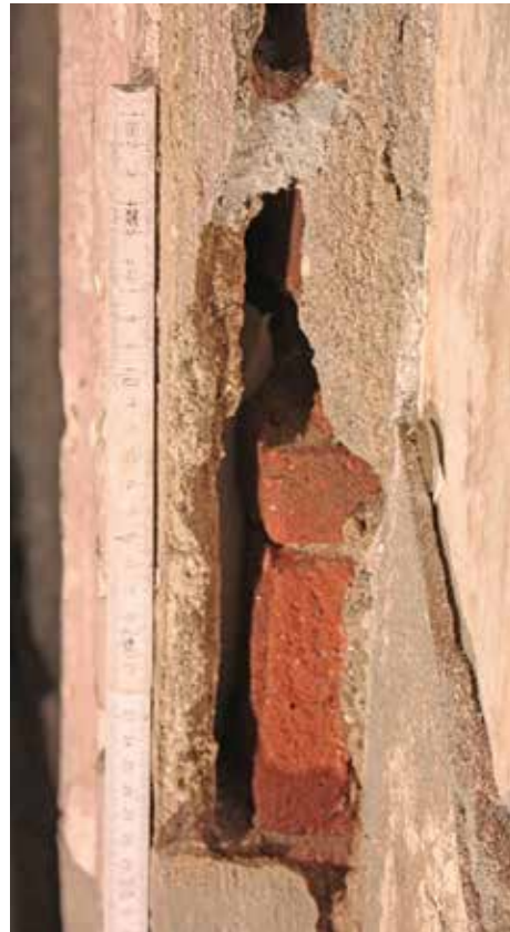
Figure 4: Delaminated pilaster in San Vincenzo Oratory, north wall
