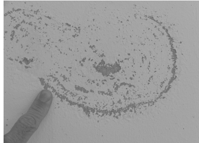
Figure 3.10 Damage pattern originating probably from the application technique (St. Nicholas church in Brouwershaven, the Netherlands)
