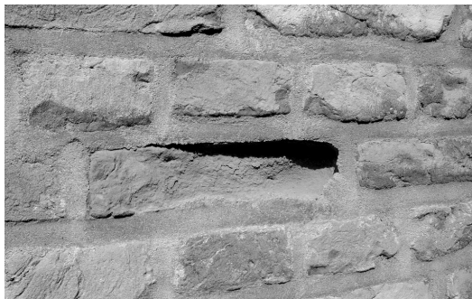
Figure 4.3 (left) Powdering of brick (exterior)
