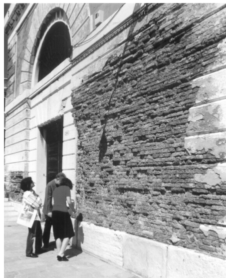
Figure 3.19 Salt damage on the exterior wall of a building used as salt storage in the past (Magazzini del sale, Venezia, Italy)
