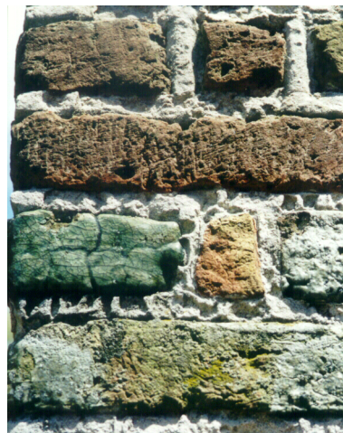
Figure 3.7 (left) Spalling of the treated outer layer of the bricks due to the application of a water repellent (building in Rotterdam, the Netherlands)
