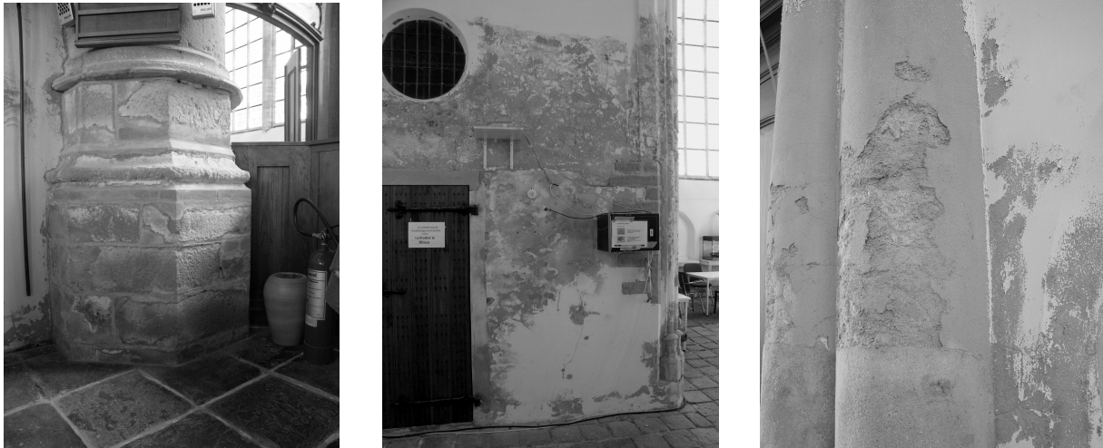
Figure 4.5 (left) Stone basements of the column showing white salt patina and sanding
