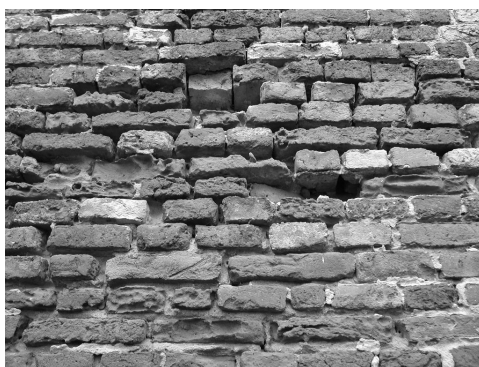
Figure 3.1 (left) Different seriousness of salt damage in bricks exposed to the same environmental conditions (church in Oostkapelle, The Netherlands)
