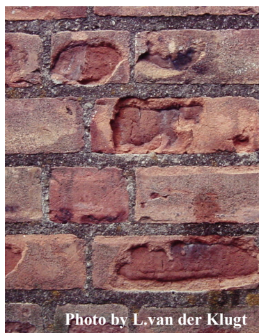
Figure 3.7 (left) Spalling of the treated outer layer of the bricks due to the application of a water repellent (building in Rotterdam, the Netherlands)
