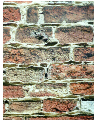
Figure 3.7 (left) Spalling of the treated outer layer of the bricks due to the application of a water repellent (building in Rotterdam, the Netherlands)
