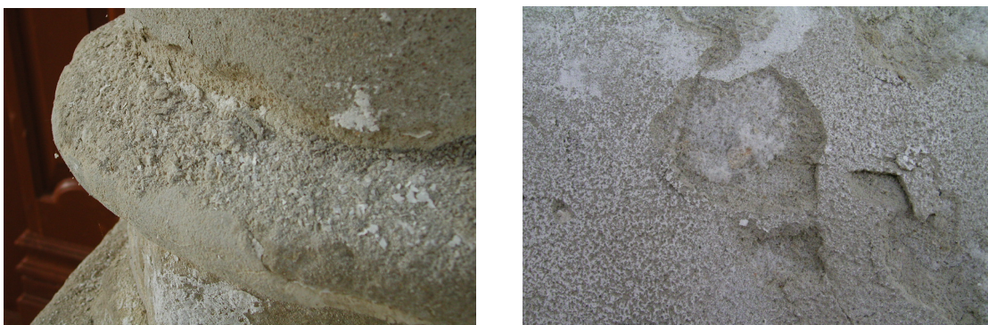
Figure 3.21 Sanding (left) and scaling (right) of the plaster (St. Nicholas church in Brouwershaven, the Netherlands)
