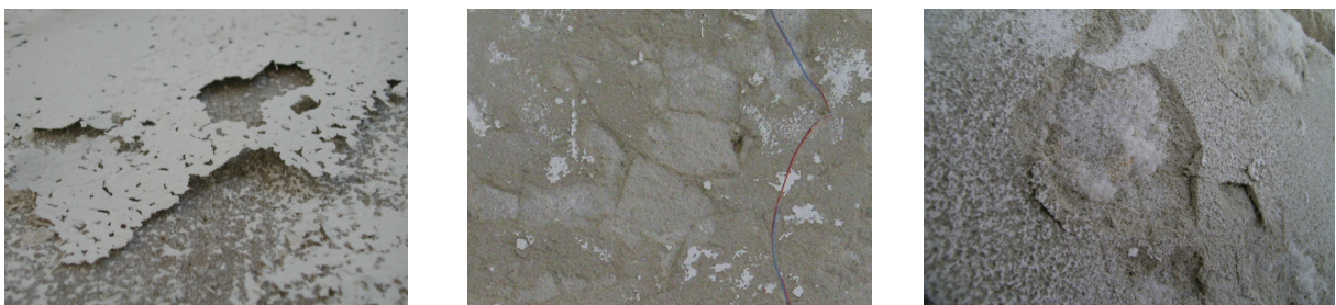
Figure 4.8 Evolution of the damage: from peeling of the paint (left), to appearance of cracks in the plaster (middle) to sanding, scaling and crumbling of the plaster layer (right)
