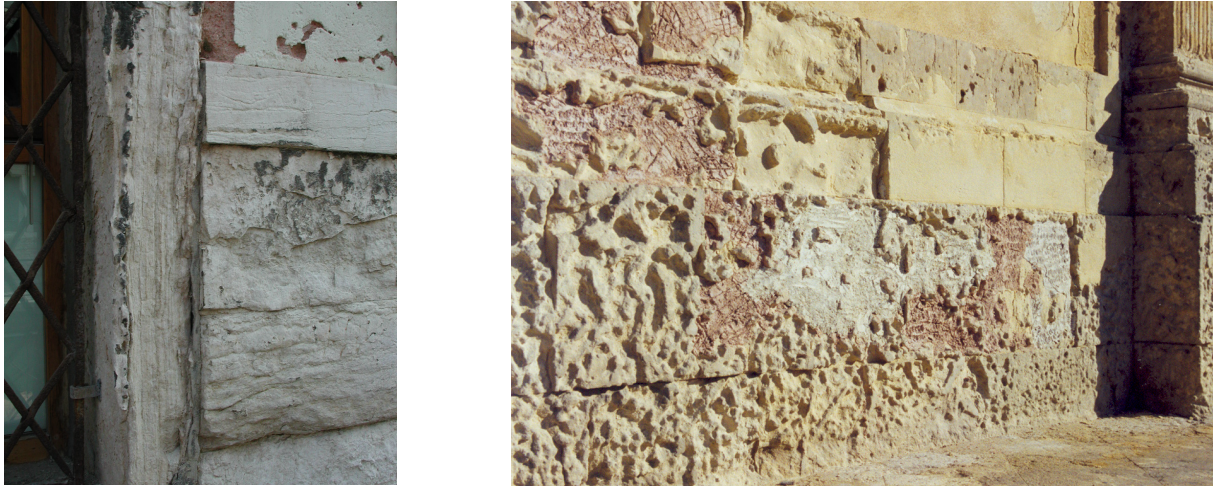
Figure 3.3 (left) Preferential weathering showing as delamination in Istria stone (building in Venice, Italy)
