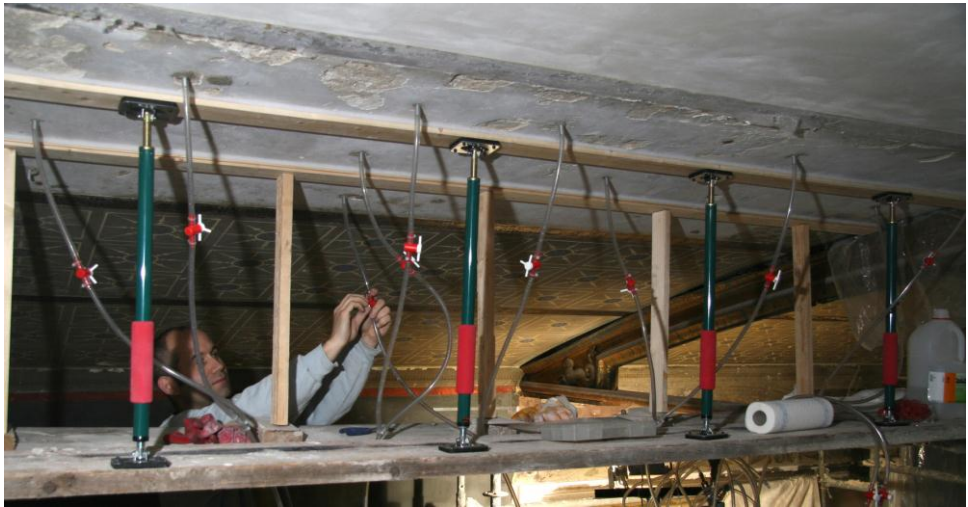
Figure 5: Installation of the hose and packer system (photo: Hüttich).
