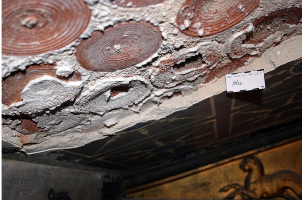
Figure 2: Massive salt efflorescence under the fallen ceiling area.
