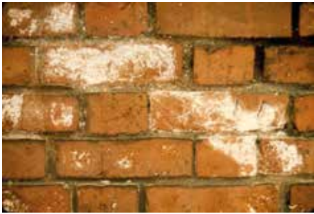
Figure 2: Detail of the brick wall showing the gypsum efflorescence formed on the parallel wall below grade to that seen in the garden at right.
