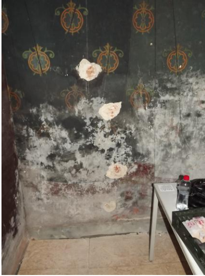
Figure 4: typical damage pattern of a 19 th century mural painting in the St-Vincentius Chapel.
