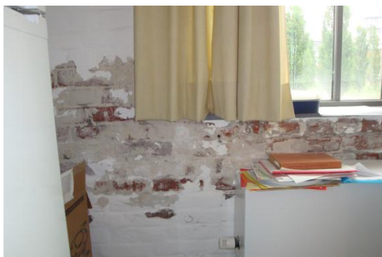
Figure 2: interior wall with salt damage due to the presence of up to 7.5 w% sodium chloride in the mortar and at least 1 w% in the brick
