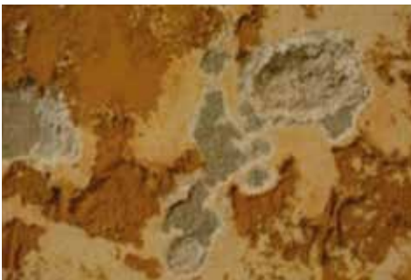
Photo 1: Deterioration of the inner walls due to salt crystallisation at Hagia Sophia, Istanbul, Turkey
